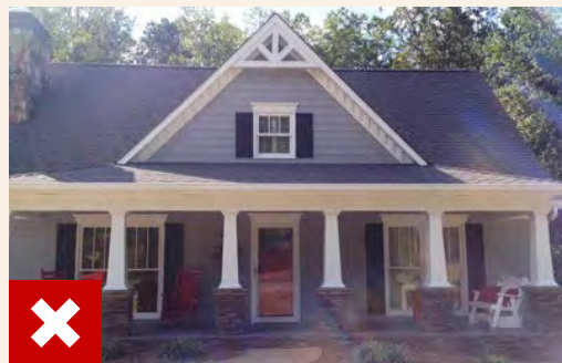
Inappropriate Column Placement: No Window Bay definition
