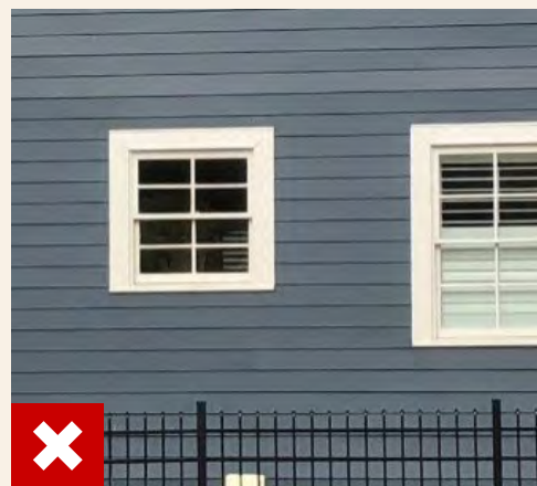
Inappropriate Window Configurations
