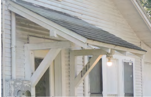
Wood Entry Door Canopy
