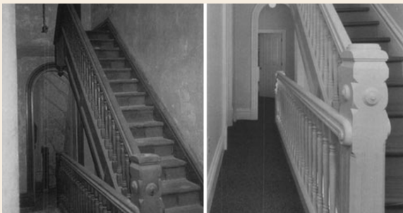
PHOTO: A large-scale historic rehabilitation project incorporated sensitive lead-hazard reduction measures. Interior walls and woodwork were cleaned, repaired, and repainted and compatible new floor coverings added. The total project was economically sound and undertaken in a careful manner that preserved the building's historic character. Before:left, after:right. Photos: Landmarks Design Associates
