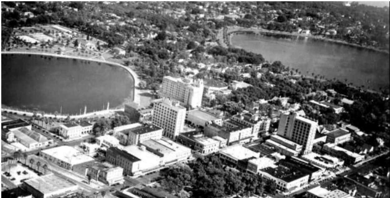
Aerial Image of Downtown Lakeland, date unknown
