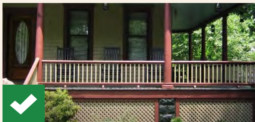
Historically Correct Handrail Height
