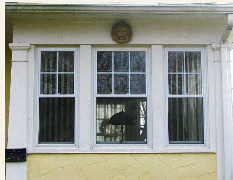
Replacement windows with four over one glazing configuration
