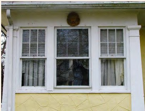
Original wood windows with six over one glazing configuration
