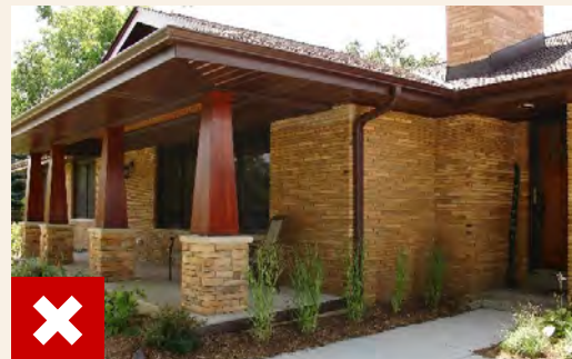
Inappropriate Porch Columns and Beam Details
