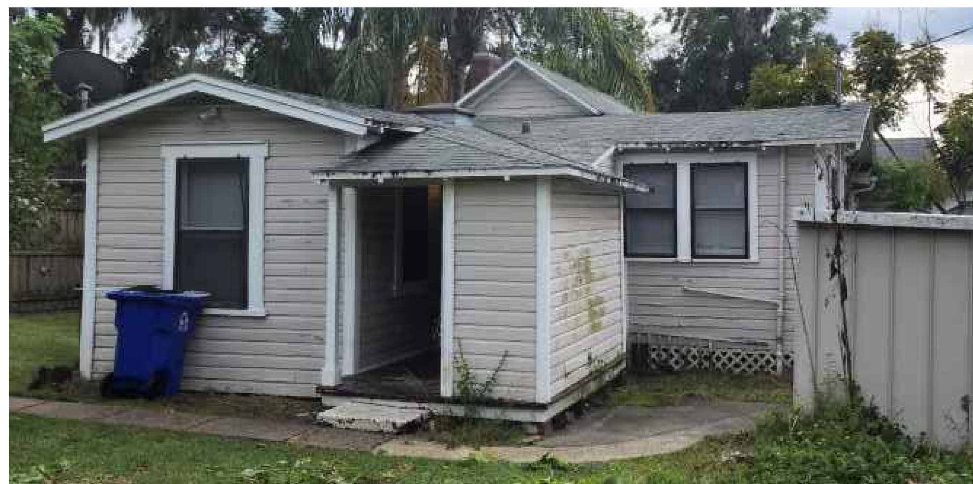
EXISTING REAR IMAGE
