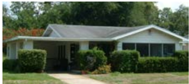
Figure 5.29: Modern Vernacular (Frame and Masonry)
