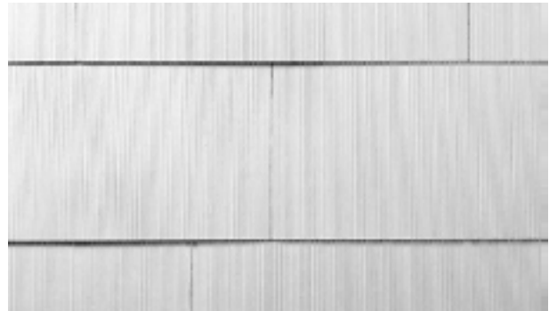
Fiber-Cement Lap Siding and/or Shingles
