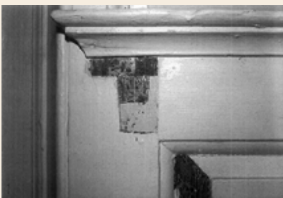
PHOTO: The paint chronology of this mantel, seen in the exposed paint layers in the left corner, proved it had been relocated from another room of the house. To remove a significant feature's paint history and the evidence of its original sequence of color by stripping off all the paint is inappropriate - and unnecessary - as part of a lead hazard reduction project. Careful surface preparation and repainting with lead-free top coats is recommended. Photo: NPS Files.
