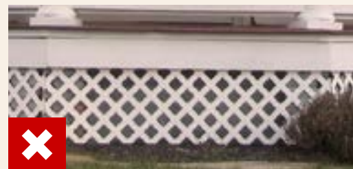
Porch Skirting Without a Frame
