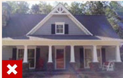
Inappropriate Column Placement: No Window Bay definition
