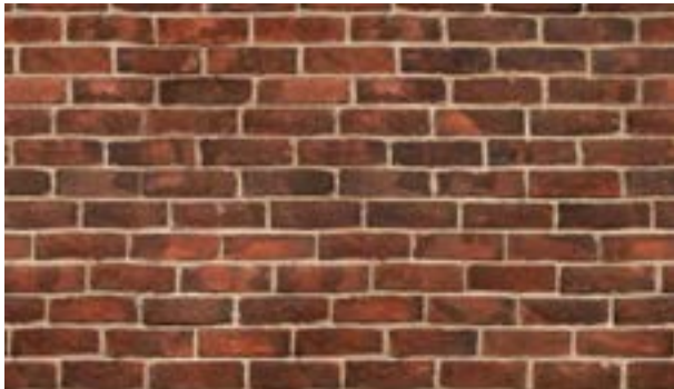
Brick Wall Surface
