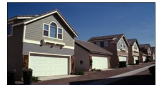
9 Units per Acre - Single Family Detached with Garage Apartment in rear of lot facing an alleyway.
