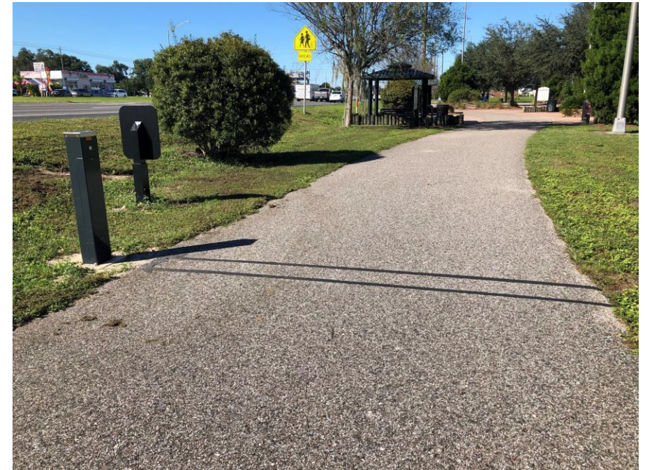
Fort Fraser Trail Counter Under Construction
