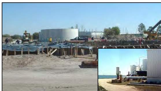
Combee Treatment Plant Under Construction
