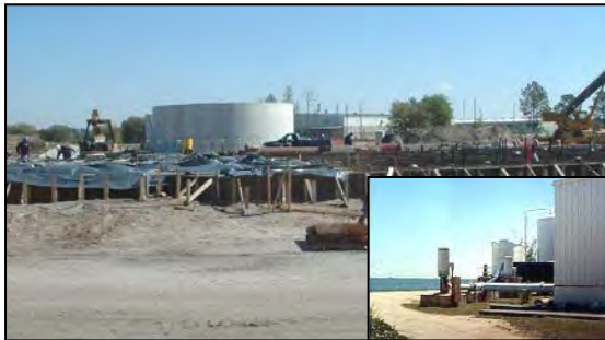
Combee Treatment Plant Under Construction
