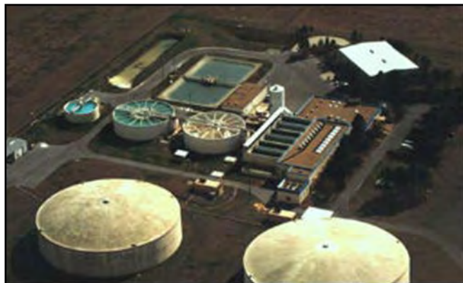
T.B. Williams Water Treatment Facility in NW Lakeland
