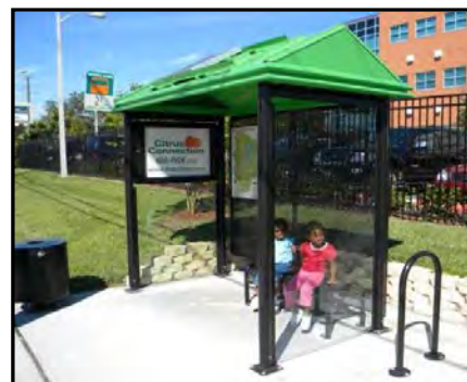
Type I Transit Shelter
