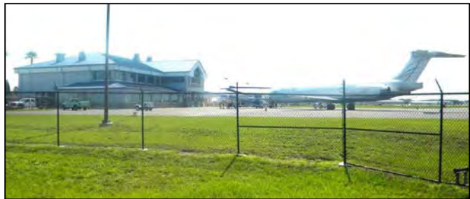
Passenger Terminal: Lakeland Linder Regional Airport
