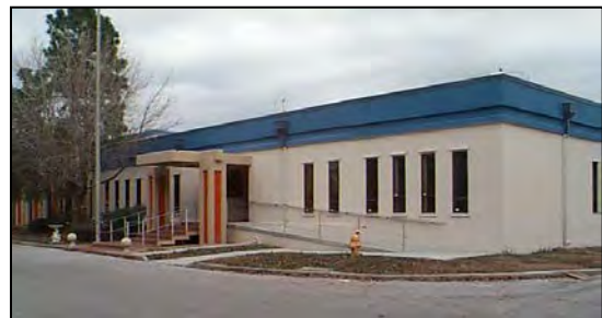
TB Williams Water Treatment Plant Administration Building
