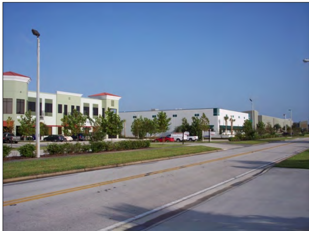
South Pipkin Road in Parkway Corporate Center
