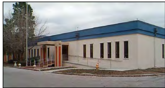
TB Williams Water Treatment Plant Administration Building
