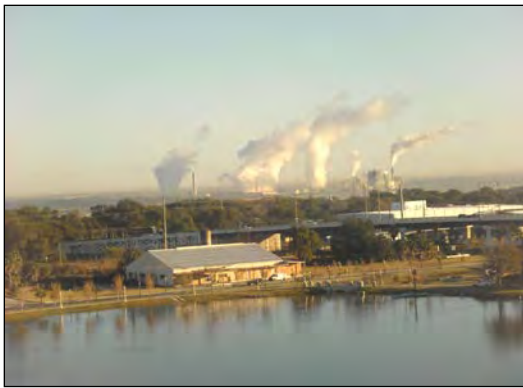
Lakeland Power Plants
