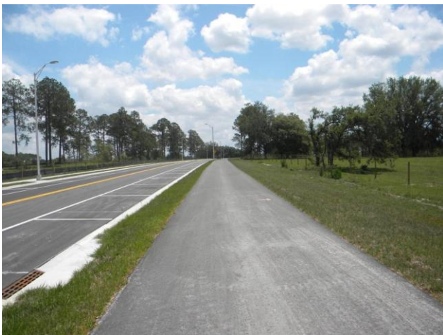
Research Way Trail at entrance to new polytechnic university currently under construction.
