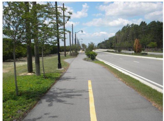
Pace Road Trail at intersection with TECO-Auburndale Trail
