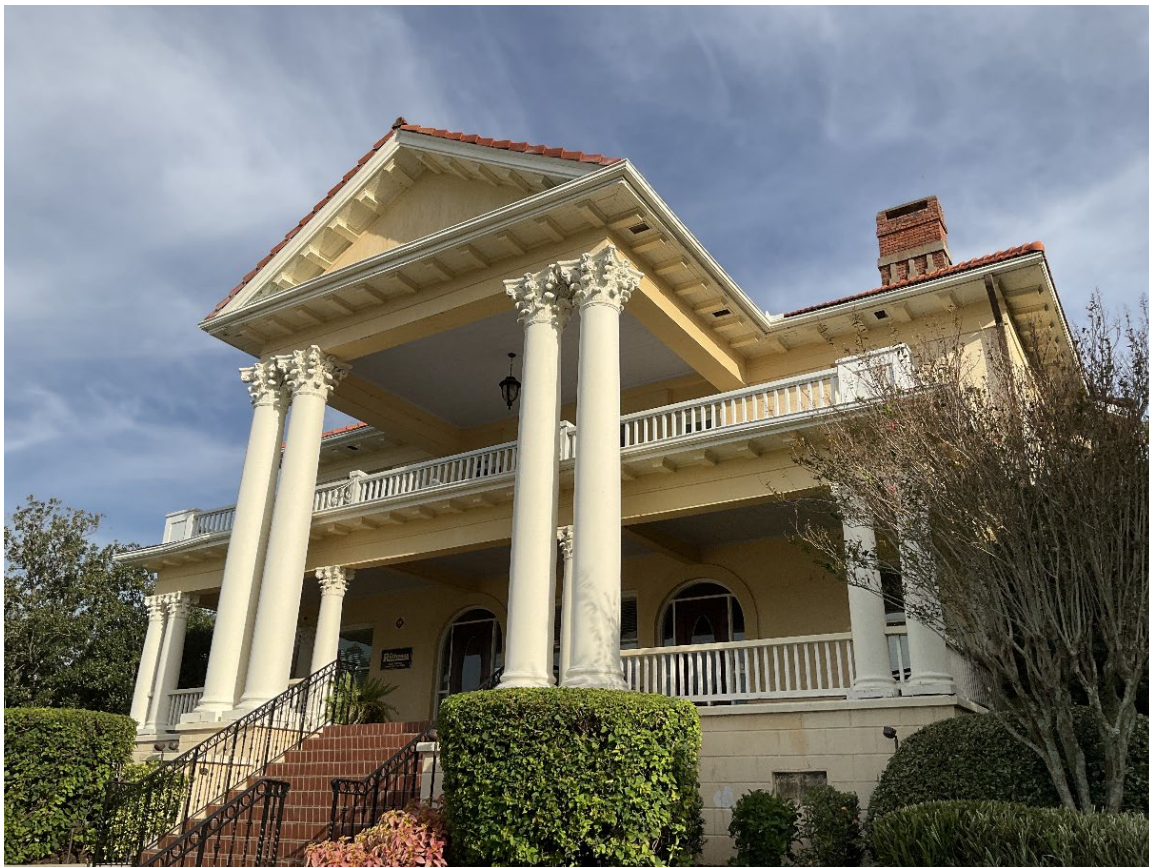
Figure 4-18. A Neoclassical Revival style building at 41 Lake Morton Drive (Ruthven Building, P003412) in the East Lake Morton Historic District.
