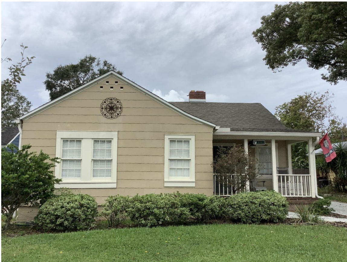
Figure 4-17. A Minimal Traditional style residence at 1017 Pennsylvania Avenue (P000856) in the South Lake Morton Historic District.
