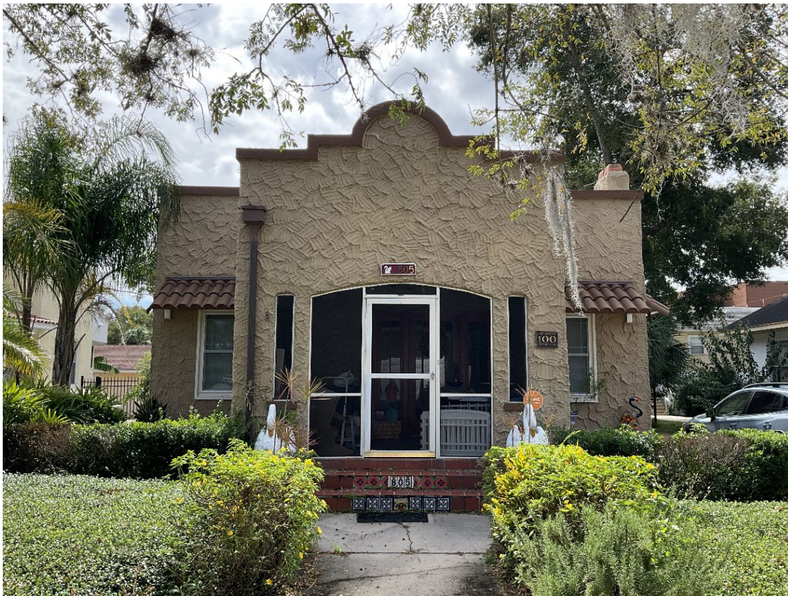
Figure 4-13. A Mediterranean Revival style residence at 805 Vistabula Street (P003461) in the East Lake Morton Historic District.
