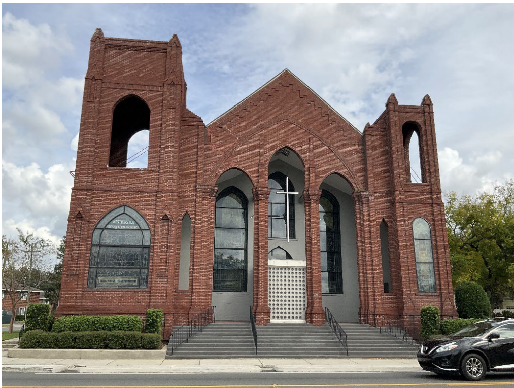
Figure 4-5. A Collegiate Gothic House of Worship at 730 S Florida Avenue (Westminster Presbyterian Church, P000562) in the South Lake Morton Historic District.
