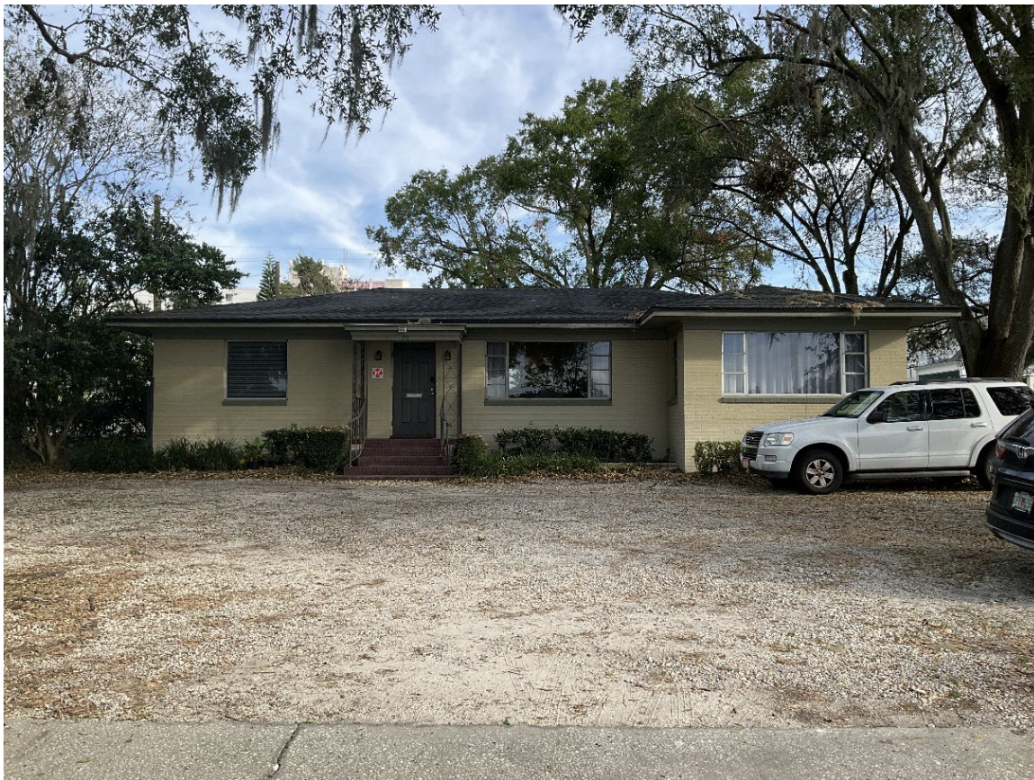
Figure 4-22. A Ranch style resource at 50 Lake Morton Drive (P009489) in the East Lake Morton Historic District.
