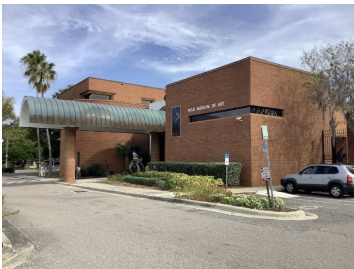
Figure 4-19. A Postmodern style building at 800 E Palmetto Street (Polk Museum of Art, P009586) in the East Lake Morton Historic District.
