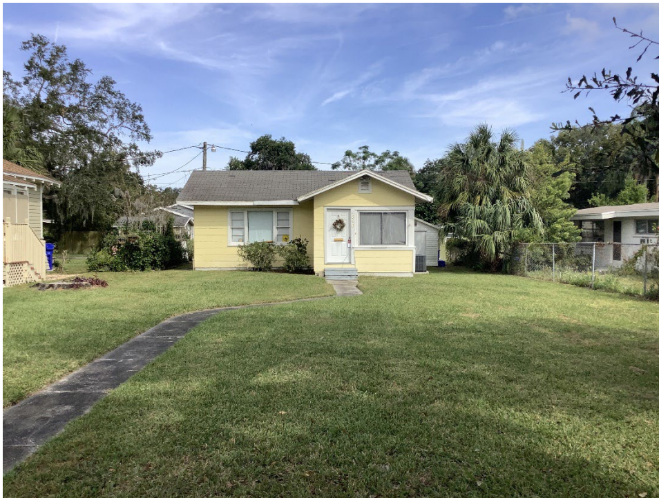
Figure 5-12. 840 E Palmetto Street (P003431) currently listed as non-contributing and recommended as contributing. Alterations to this circa 1940, Minimal Traditional style home are limited to the application of asbestos siding and the replacement of its original windows.
