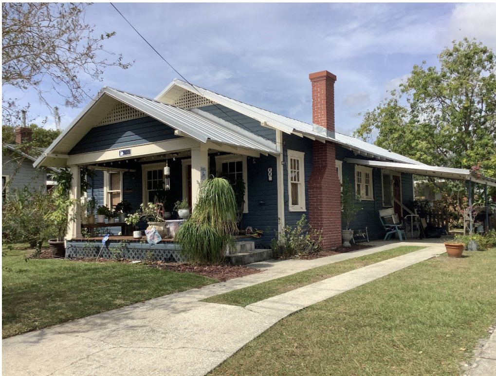
Figure 4-4. A Bungalow type residence at 840 E Walnut Street (P003514) in the East Lake Morton Historic District.
