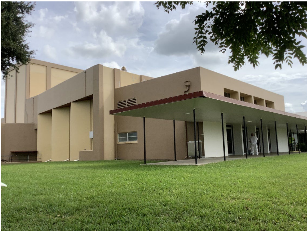
Figure 4-16. A Moderne style building at 215 S Lake Avenue building B (P009567) in the East Lake Morton Historic District.
