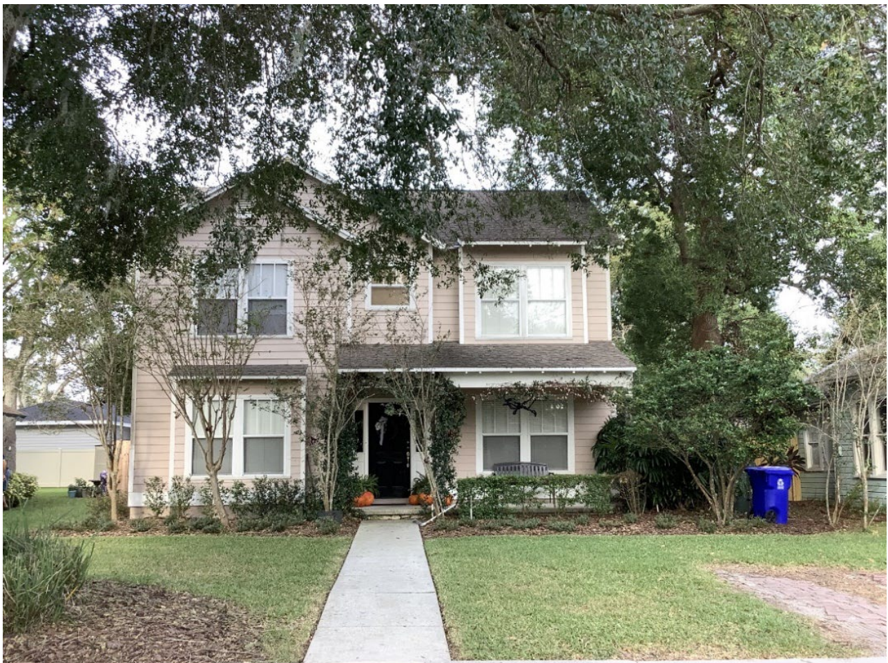
Figure 5-18. 827 S College Avenue (P000521), a previously recorded recommended non-contributing building in the South Lake Morton Historic District. This building has lost its integrity due to the large two-story addition made to its façade.
