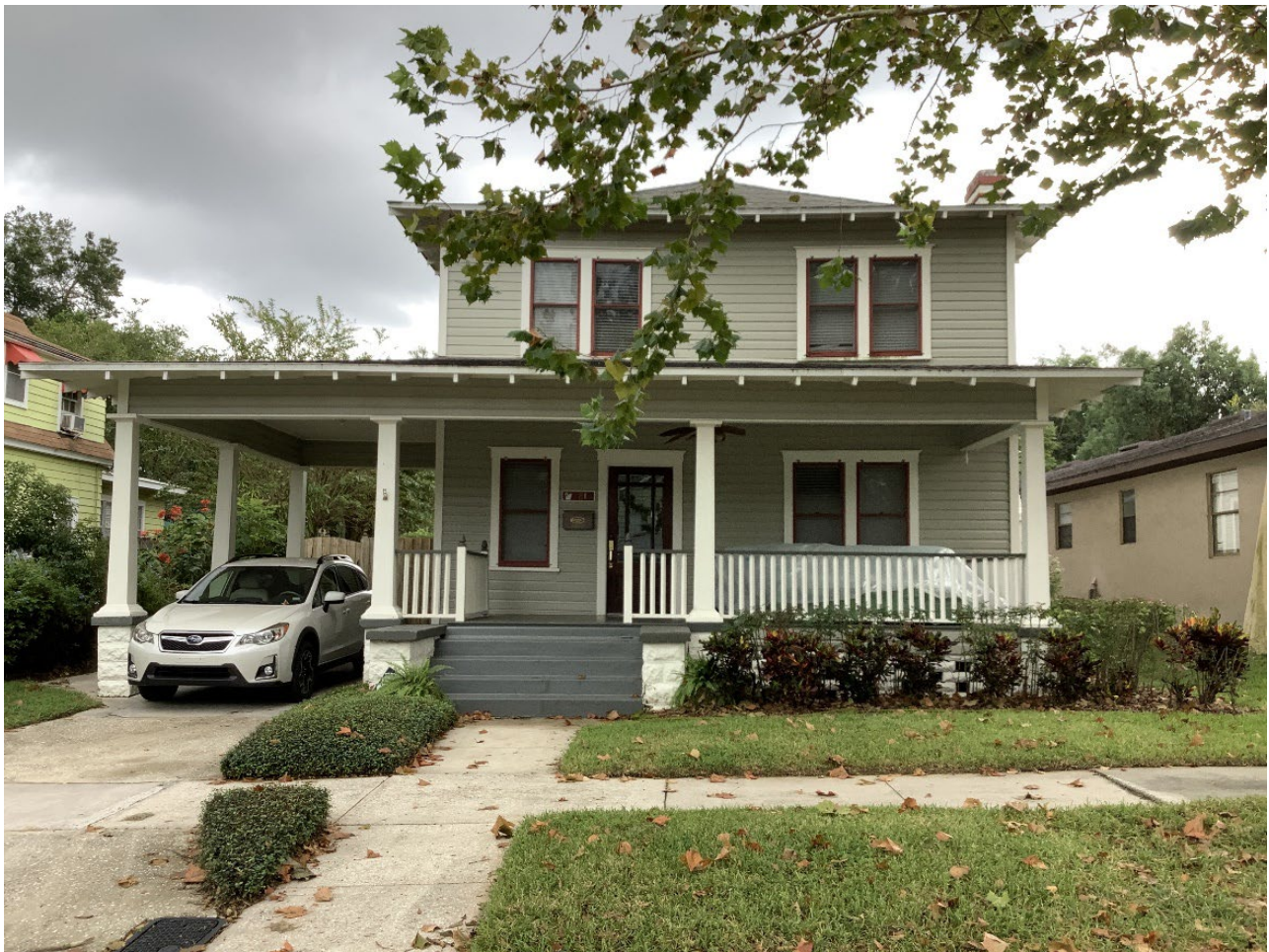
Figure 4-3. An American Foursquare style residence at 810 S Mississippi Avenue (P000694) in the South Lake Morton Historic District.
