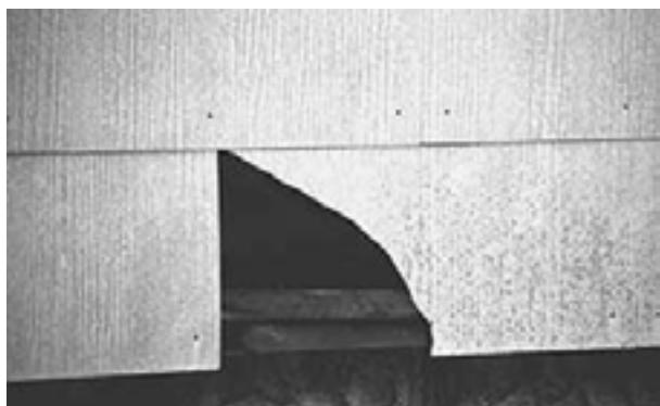
*Figure 8.5: Asbestos-cement products most commonly deteriorate by cracking and chipping. These kinds of deterioration are not typically feasible to repair, and therefore it is recommended that a non-asbestos fiber cement piece be used as a replacement (photo by author).*
