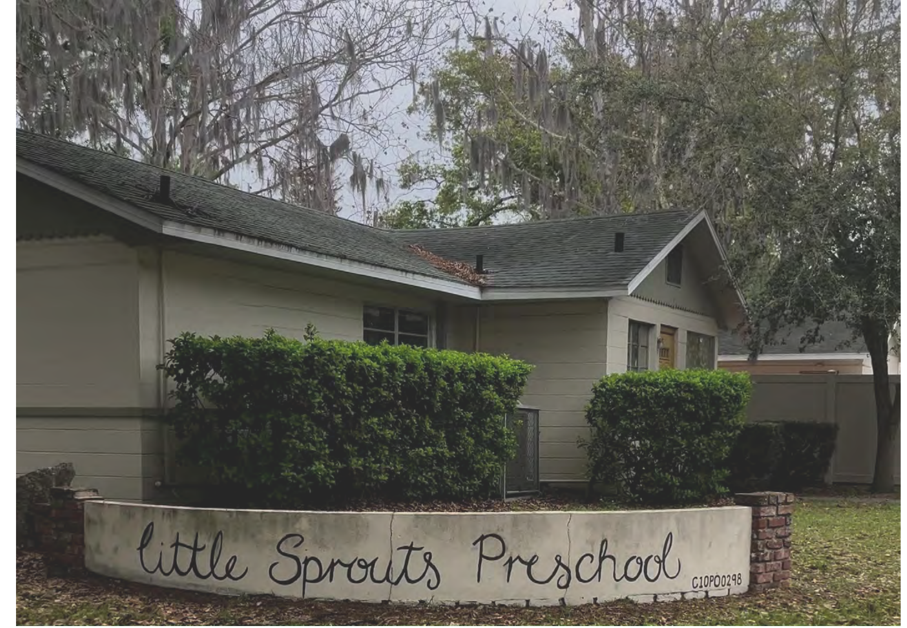
EXISTING BUILDING PHOTO - VIEW OF EXISTING MONUMENT SIGN AT SOUTHWEST CORNER OF SITE
