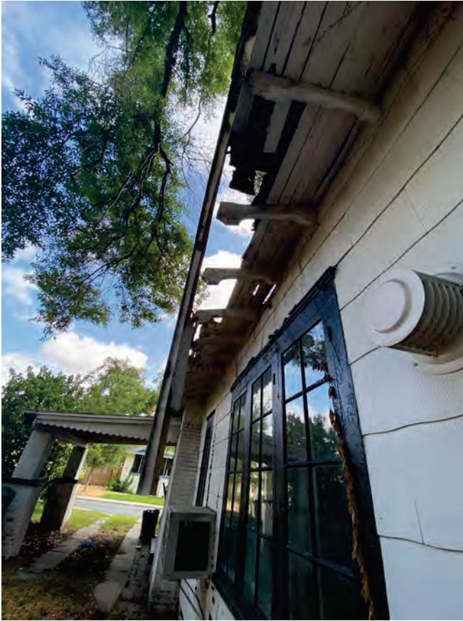
West Roof Overhang
