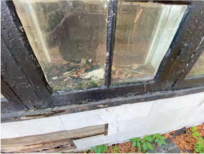
West Window Sill in Dining Room
