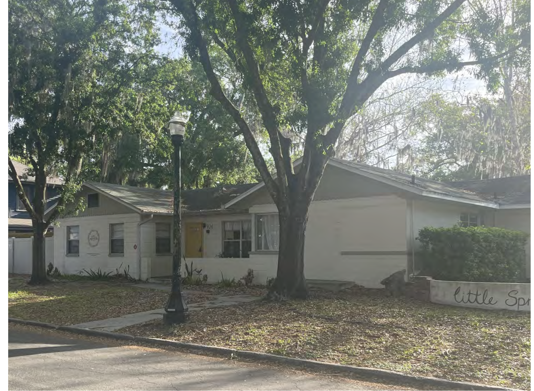
EXISTING BUILDING PHOTO - VIEW OF SOUTH SIDE OF BUILDING 1
