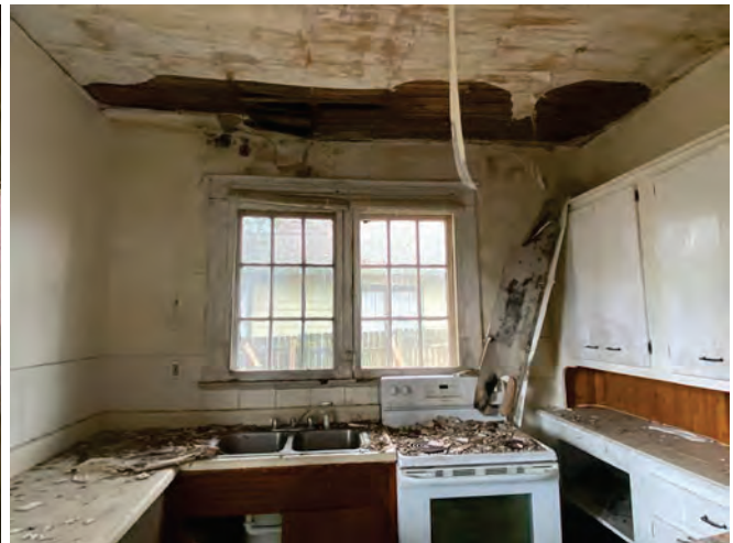
Kitchen @ Southwest Corner of the House
