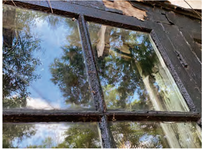
West Window Header in Dining Room
