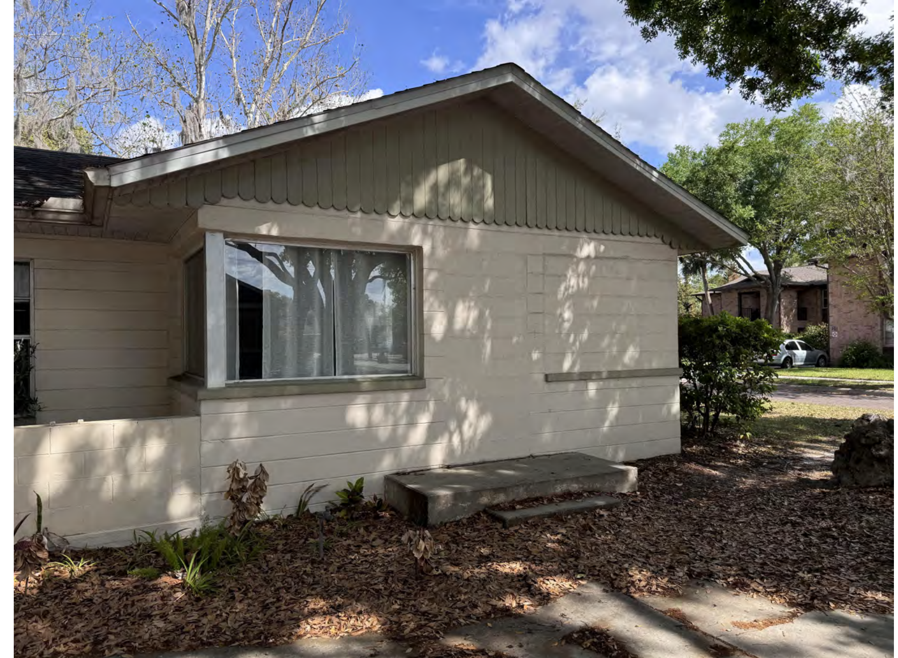
EXISTING BUILDING PHOTO - VIEW OF GABLE ROOF ENDS
