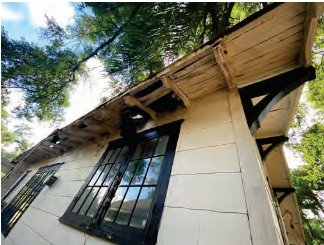
West Roof Overhang
