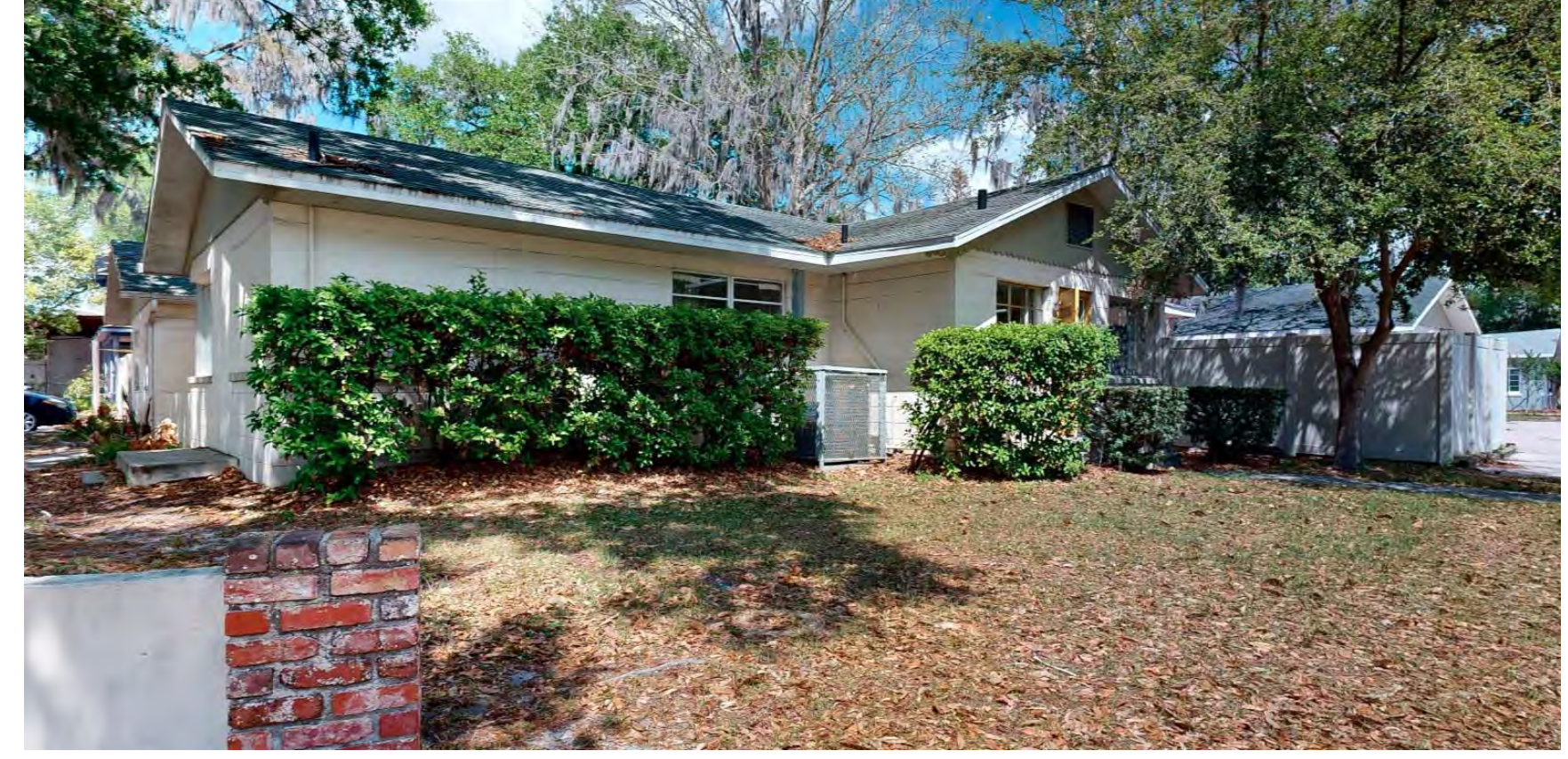
EXISTING BUILDING PHOTO - VIEW OF SOUTH SIDE OF BUILDING 1
