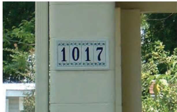
Figure 5.31: Concrete Block with Rounded Edges
