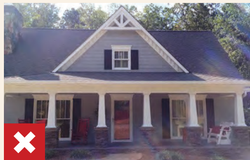
Inappropriate Column Placement: No Window Bay definition
