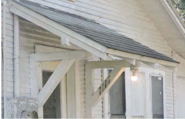
Wood Entry Door Canopy
