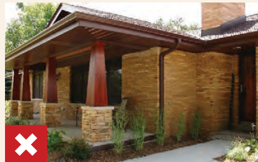
Inappropriate Porch Columns and Beam Details
