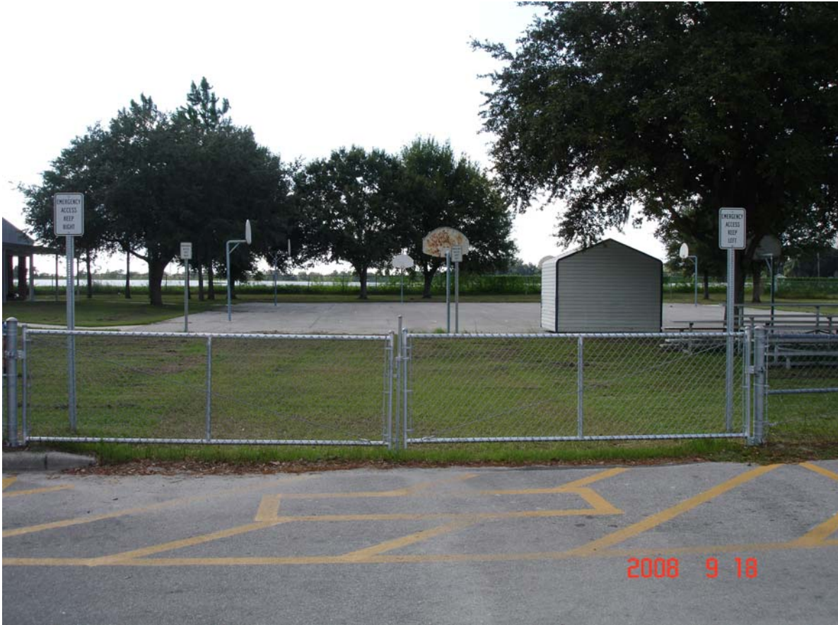
Socrum Elementary Engineered Turf installation for fire truck access through gate and between signs.
