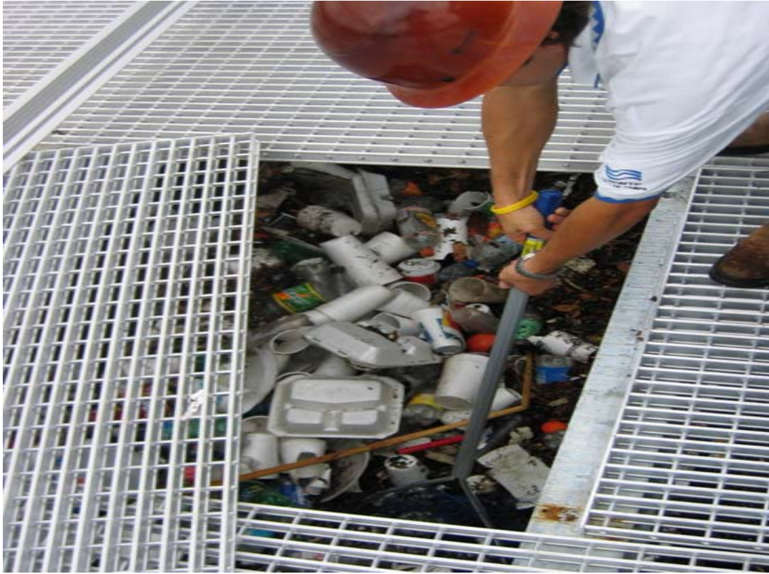
Trash Collection Basin at the Lake Parker Southwest Outfall Regional Stormwater Treatment area at Lakeshore Drive and Bon Air Street., Lakeland, FL.
